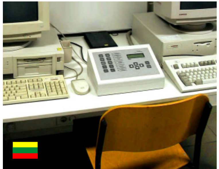
BAE used in local point heating control room Lithuania
