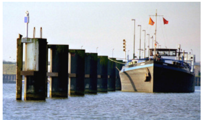
LEDFORCE self-contained on pier (NL)
