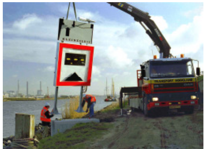
Erection of Depth Indication Display Sign (Ijmuiden, the Netherlands)
